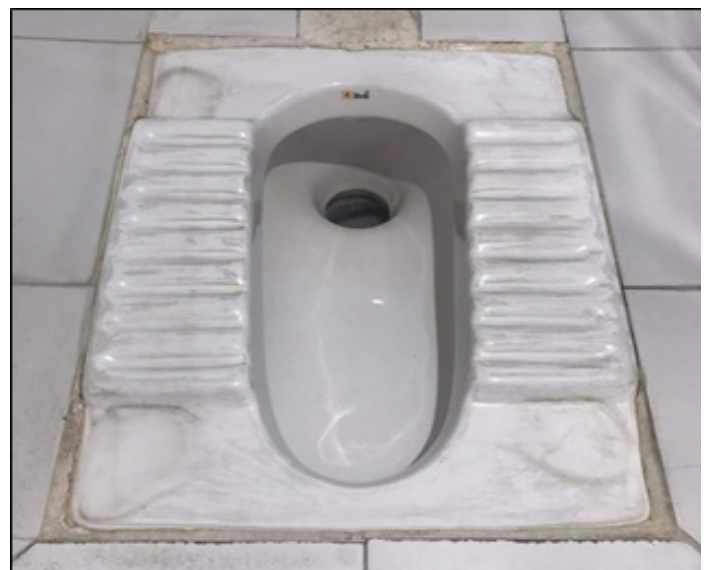
Figure 1. Floor leveled squat toilet
